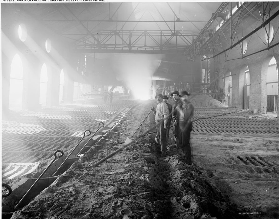
Casting pig iron, Iroquois smelter, Chicago 1890
